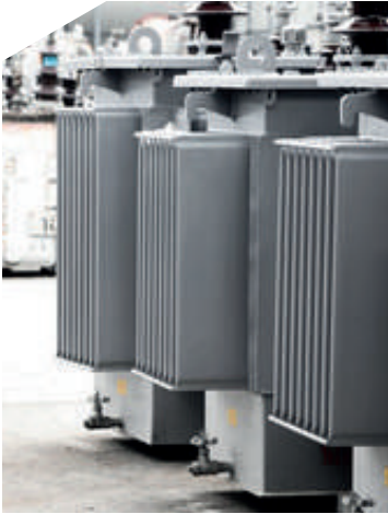
Transport of current transformer
